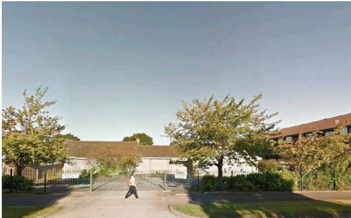
photograph of view 3; looking towards existing site entrance
