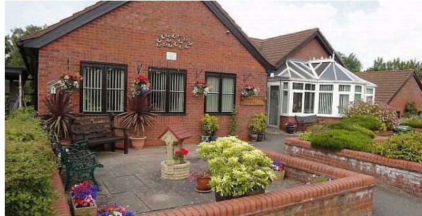
Case 5: Crescent Crofts self-managed 'very sheltered hsg' West Midlands
