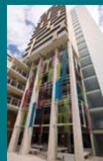
Front Cover: LHA-ASRA Elmgrove Point, Plumstead
