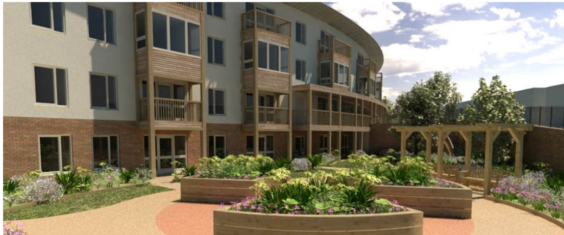
The external view of extra care scheme: Ravensfield, Dukinfield
