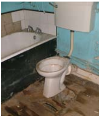
Bathroom before and after renovation
