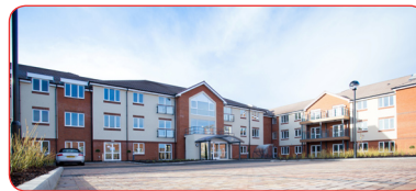
New Fortis Living development in Worcester
