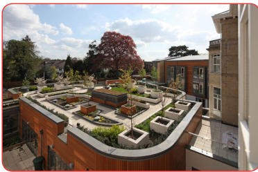
Accessible roof garden at James Terry Court, Croydon
