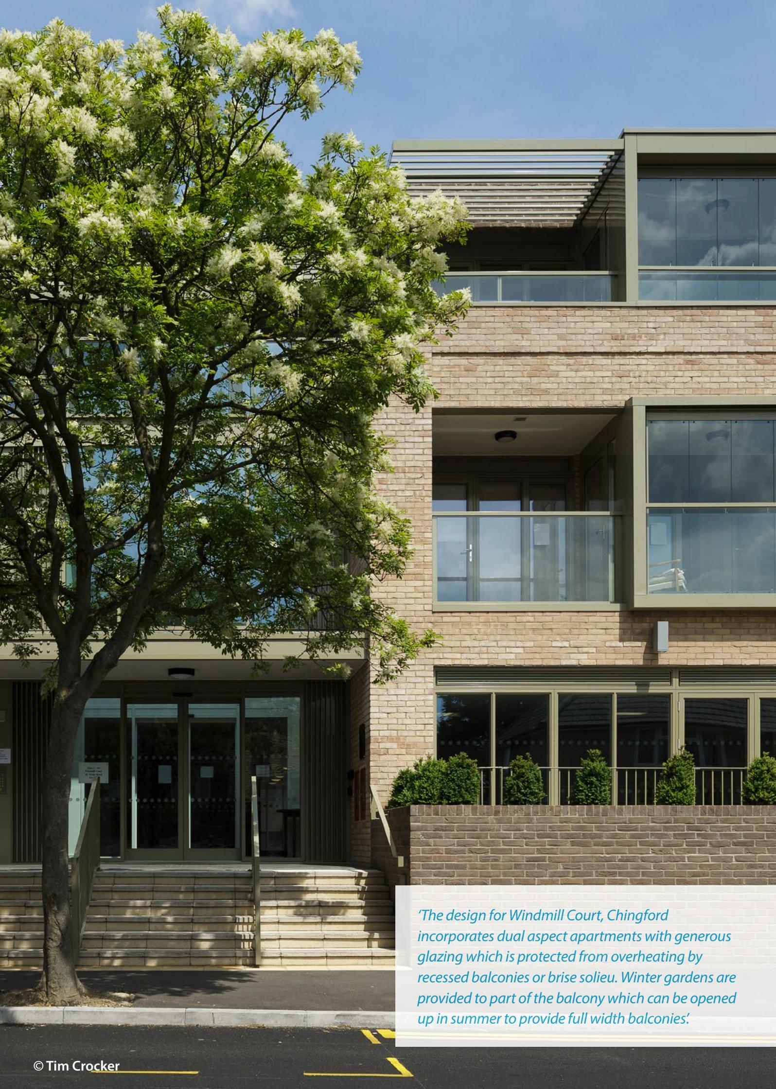
*'The design for Windmill Court, Chingford incorporates dual aspect apartments with generous glazing which is protected from overheating by recessed balconies or brise solieu. Winter gardens are provided to part of the balcony which can be opened up in summer to provide full width balconies.'*
