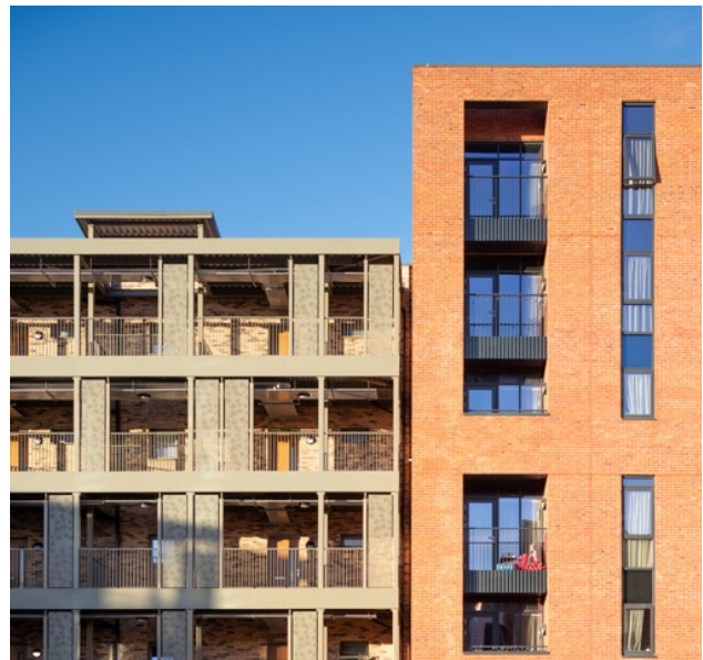
Bowes House: HAPPI-informed homes for independent living at The Depot
