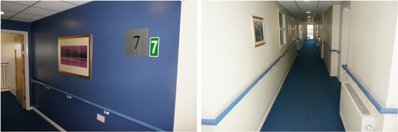
Dementia-friendly design: Corridors are colour-coded to tell people what floor they're on
