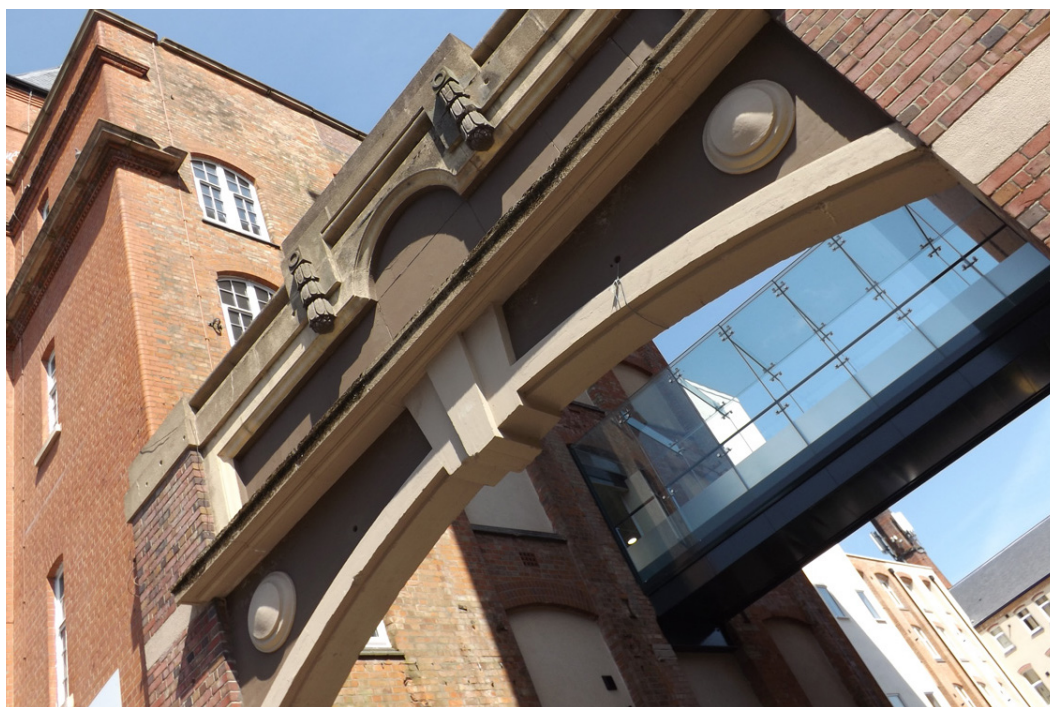
The two schemes are joined by a first-floor corridor
