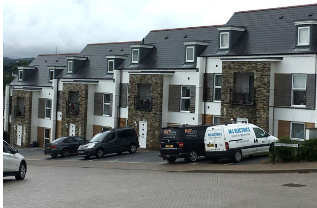
Tregorrick Way, St Austell, outside of the four ground floor block
