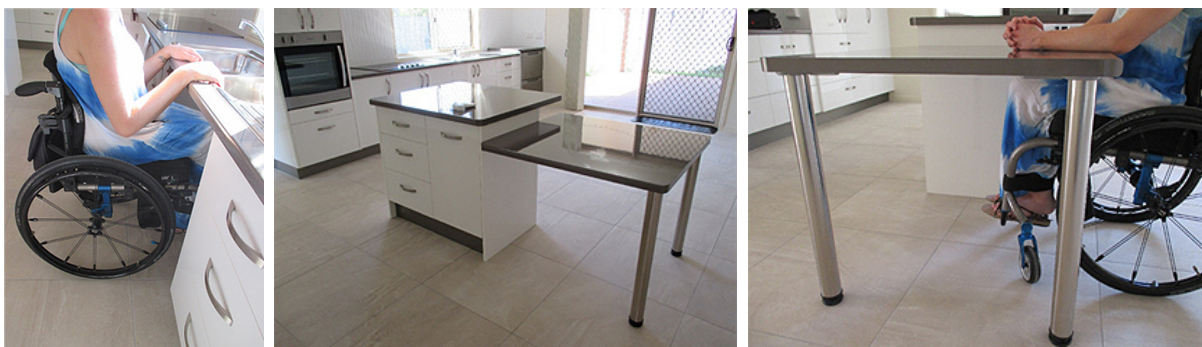
Kitchen modifications for wheelchair users
