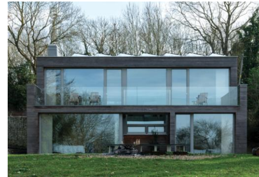
Lark Rise, Chiltern Hills. Passivhaus Plus certified. © Bere:architects
