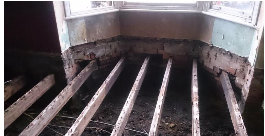
Achieving airtightness is possible in retrofit, but it is often necessary to strip back to the basic structure and perform basic repair work before methodically applying airtightness products and principles. Always consider risk of moisture and condensation.
