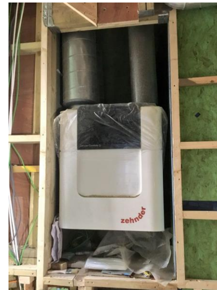
Image of Zehnder MVHR unit being retrofitted into an existing house (© Bowtie construction)
