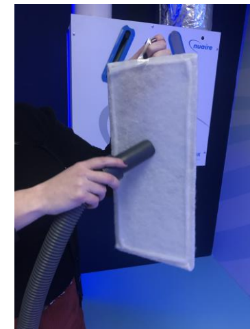
MVHR filters are easy to remove and clean, clean filters improve energy efficiency
