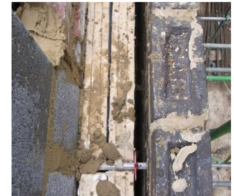
Left: an example of good Expanded Polystyrene insulation installation. Right: An example of poorly installed partial cavity installation, loosely fitting, and cement dropped atop and inside cavity.
