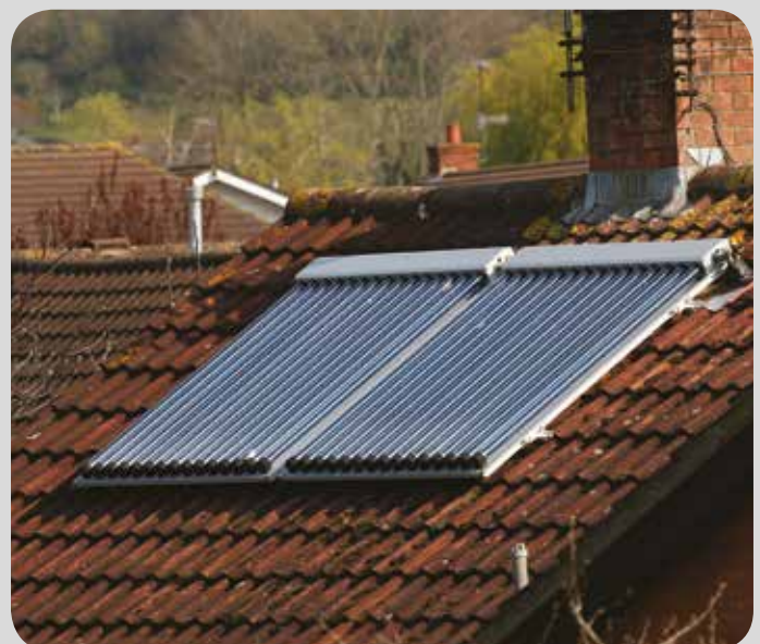
Roof space can be used for solar hot water panels
