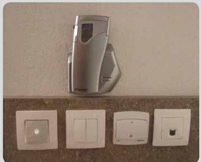
Temperature, light and ventilation controls in flats
