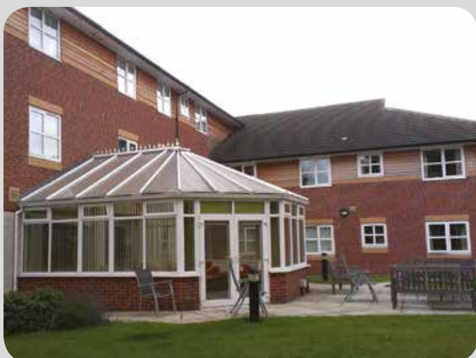
A typical modern care home building
