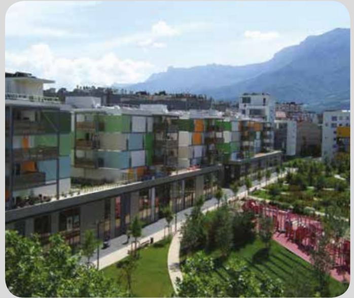
The case study apartments in Grenoble
