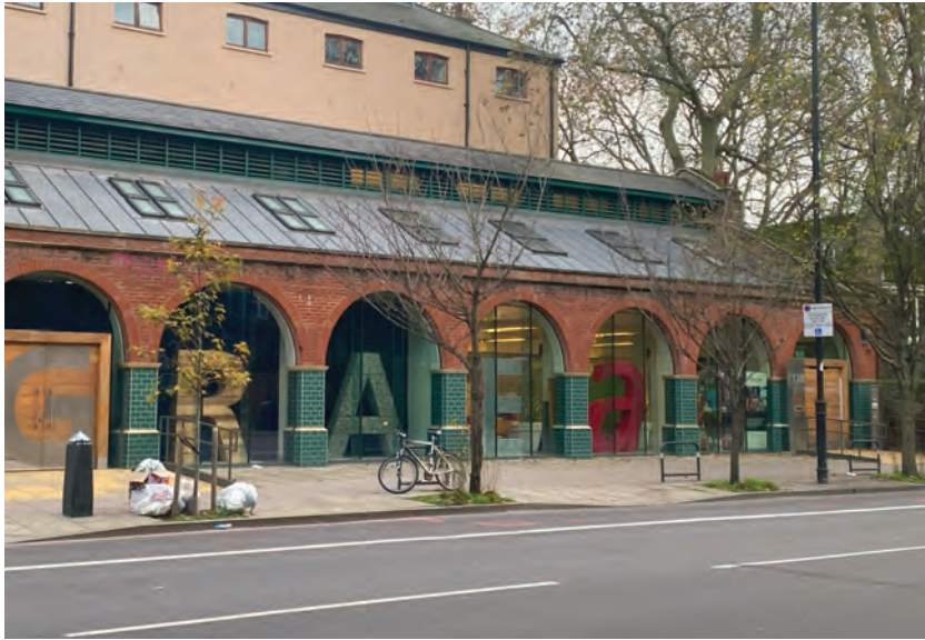
Exterior view of Graeae, Bradbury Studios London. Designed by Artillery Architecture & Interior Design and Paragon Management. Photo: Jos Boys.
