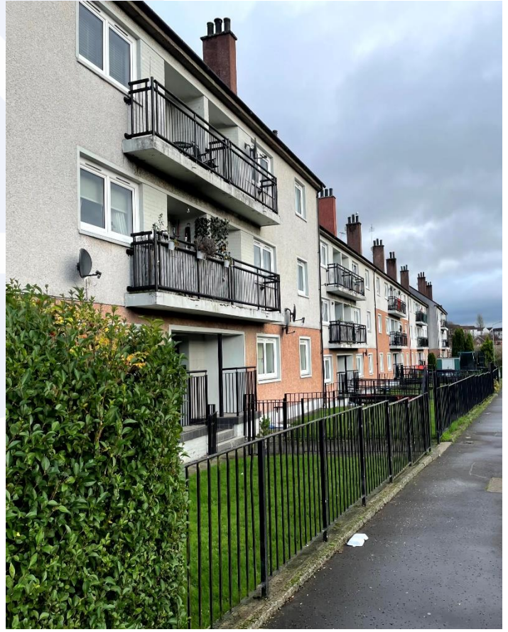
Figure 7: 1950s tenemental rehab (source: McKee)
