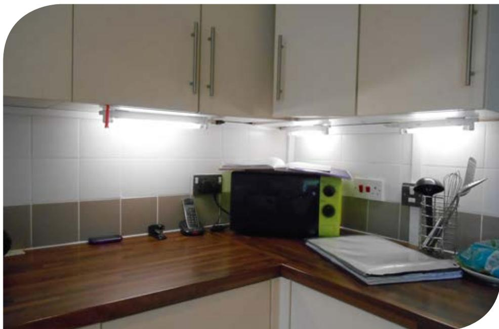
**The photograph displays unshielded task lighting that is emitting glare in a kitchen of a supported housing scheme for tenants with learning disabilities and sight loss. Unfortunately, this potentially beneficial lighting feature cannot be switched on as one of the tenants find that the glare causes them pain. Fitting a pelmet at the base of the wall unit would shield the glare and potentially alleviate this issue and enable tenants to benefit from this lighting feature.**
