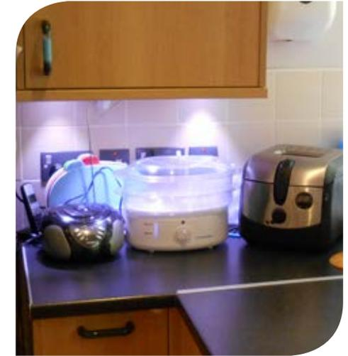
The photographs display task lighting fitted under the kitchen wall units in a supported housing scheme for people with learning disabilities and sight loss. A pelmet has been used to ensure that the under cupboard lighting cannot be viewed directly.
