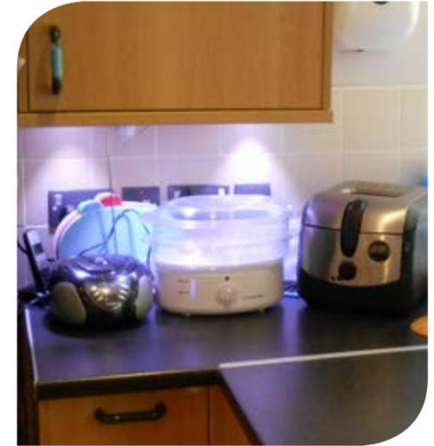
The photographs display task lighting fitted under the kitchen wall units in a supported housing scheme for people with learning disabilities and sight loss. A pelmet has been used to ensure that the under cupboard lighting cannot be viewed directly.
