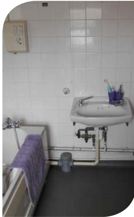
**Bathroom in a supported housing scheme. The bathroom has no contrast between the sanitary ware, grab rails and white tiles. The tiles are a gloss finish which is causing glare and reflections (see Sections 3.3.5 and 3.5).**
