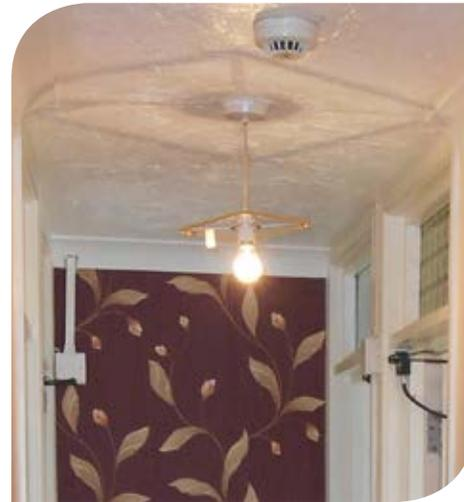
Glare is being emitted from the undiffused light. The issue is made worse by the application of satin paint which is causing pools of light on the wall (see Section 3.5). Fitting the light with a cost effective paper globe shade would help distribute the light and diffuse the lighting. Using a matt paint would prevent the pooling of light on the wall.
