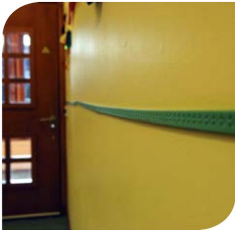
**A tactile marker has been placed along a corridor to aid trailing and support wayfinding.**
