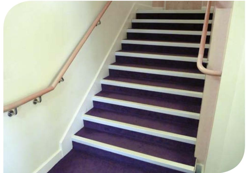
**Edge of steps on stairs highlighted by contrasting nosings and handrail highlighted by a colour that clearly contrasts with the wall. The colour contrasted nosing that wraps around both the tread and the riser of the step is an excellent feature that clearly highlights the position of the edge of the step against the carpet. This assists people in locating the edge of the steps when going up and down the stairs.**
