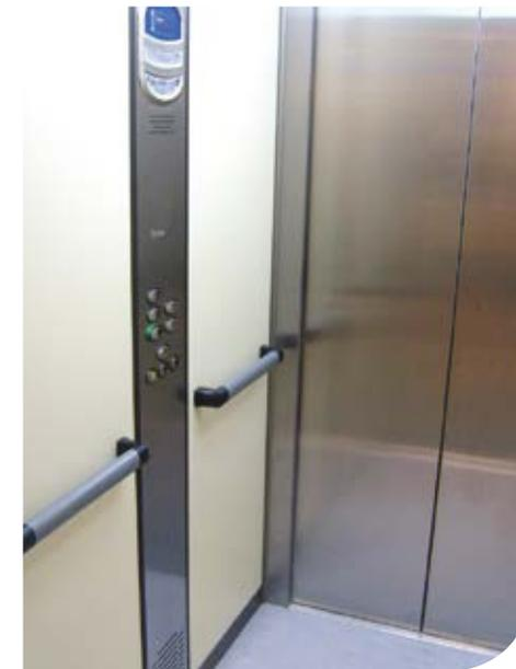
**Some individuals did not like to use the lift in the photograph on the right hand side due to large amount of reflective surfaces and full height mirror. A selection of matt finish for the walls is recommended as displayed in the following image.**
