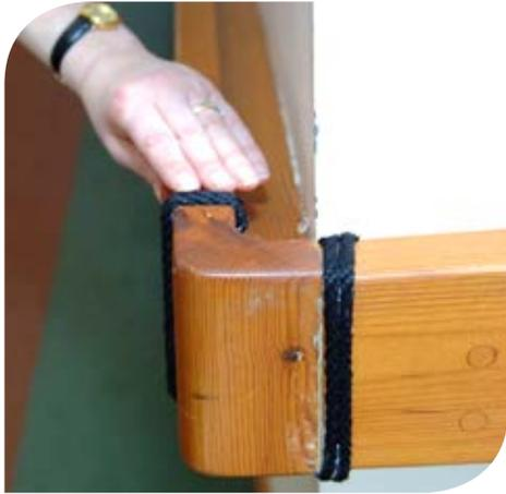
**A rope has been placed on the end of the handrail to act as a tactile marker and indicate a change of direction.**
