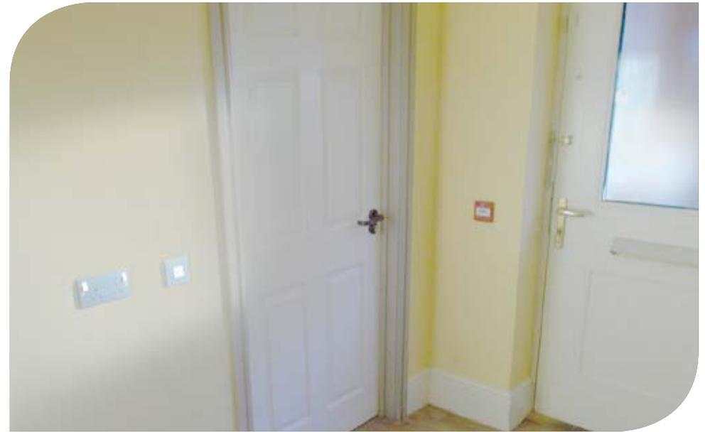
**In this supported living scheme for tenants with learning disabilities and sight loss, the housing association has specified colour contrasted D shaped lever handles. They have used a dark architrave to highlight the position of the door.**
