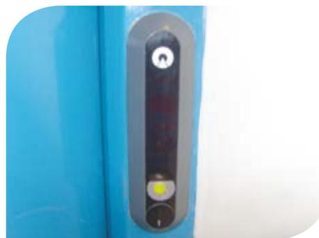
**The addition of a green coloured bump-on is used to help the buildings users to locate the lift button against its background.**
