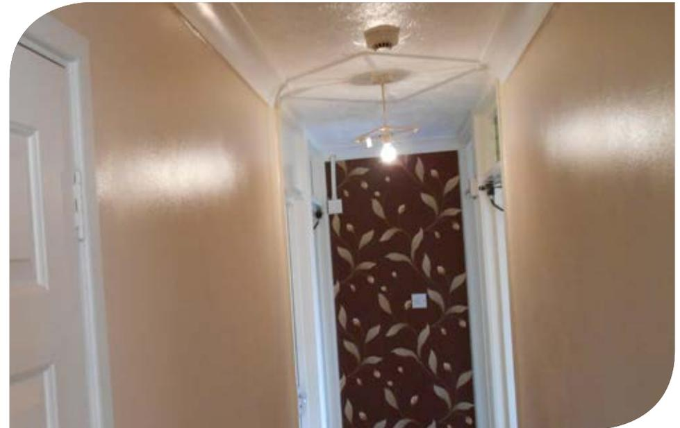
**Pools of light on wall caused by the use of a satin paint finish. The patterned finish on the wall at the end of the corridor could cause confusion.**
