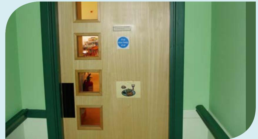
**The leading edge of the door has been painted to contrast against the face of the door to highlight the position of the door when it is open.**
