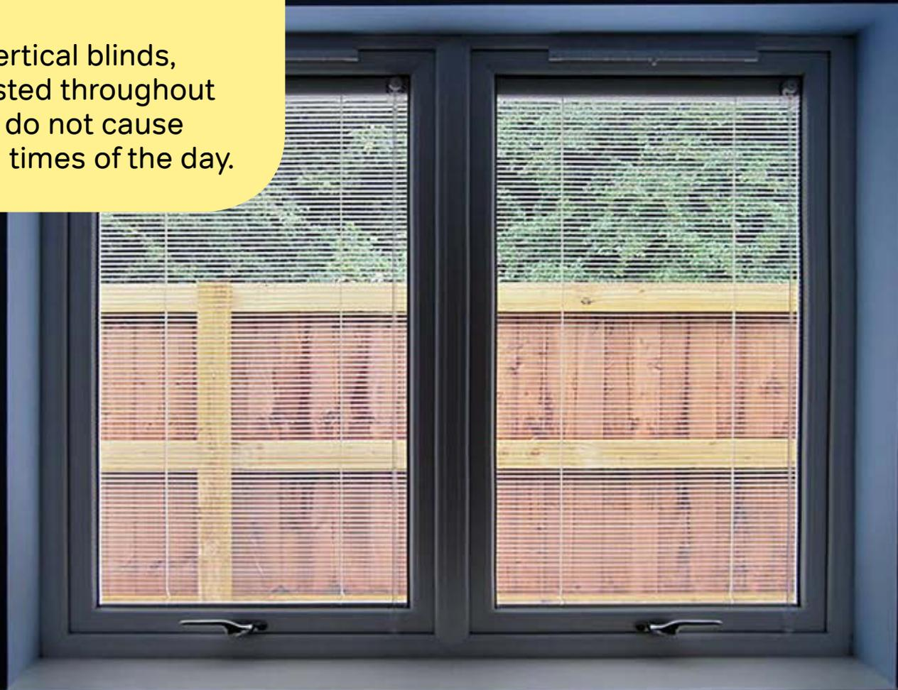
**Window fitted with integral blind in a kitchen of a supported living scheme for tenants with learning disabilities and sight loss. The blind enables tenants to control natural lighting and glare to meet their individual lighting needs.**
