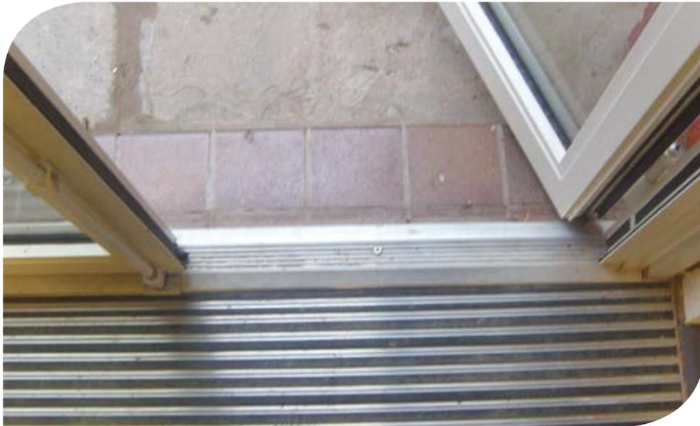
**Threshold strips at entrances to buildings can often be trip hazards and a barrier for wheelchair users. In new buildings, and when refurbishing or maintaining housing, we recommend level thresholds in accordance with the recommendations within Part M and BS8300 (BSI 2009+A1:2010).**
