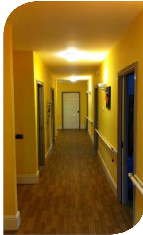
**The photographs display a fully contrasted corridor in a supported housing scheme for tenants with learning disabilities and sight loss. Flooring, wall and ceiling finishes have been selected to ensure that wall, floors and ceilings contrast. The doors have been highlighted by a contrasting architrave. Walls, floors, ceilings and doors are highlighted even when the lighting is switched off and the corridor is lit by a light tunnel.**
