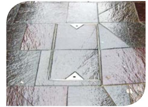
**Manholes can be perceived as obstructions or holes. A manhole cover in the same material as the paving slab would be preferable. The manhole cover in the picture on the right has been covered using the same material as the surrounding surface which is a good feature.**
