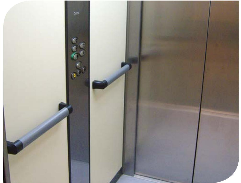
**A lift floor and wall that has been colour and tonally contrasted.**
