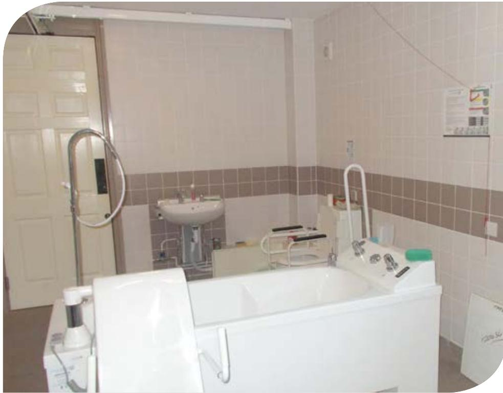
**The photographs display a bathroom in a supported housing scheme for people with learning disabilities and sight loss. The finishes of the flooring, tiles, and grab rails have been chosen to ensure the sanitary ware, grab rails and shower are highlighted against the key adjacent surfaces. In this large bathroom, a combination of two tiles have been used to highlight the position of the toilet, sink and grab rails and shower.**
