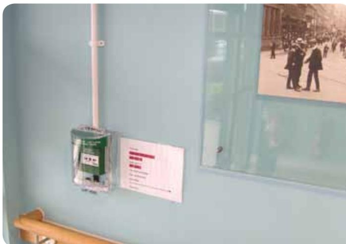
In one nursing home this problem was alleviated by covers being fitted with an alarm which sends a piercing noise when touched. This prevented residents lifting the flap on the box and opening the fire doors.
