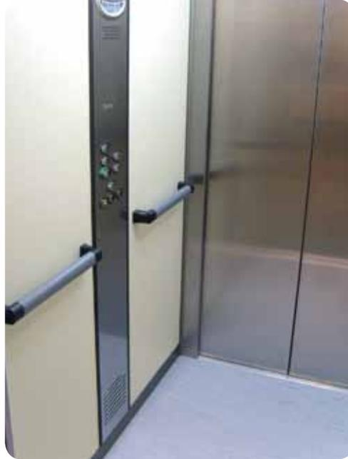
The addition of a green coloured bump-on is used to help residents with sight loss and dementia to locate the lift button against its background.
