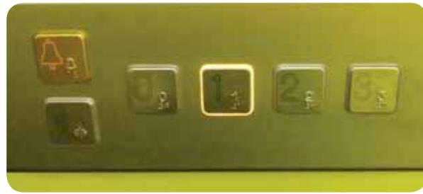
The control panels have tactile numbers and braille.
