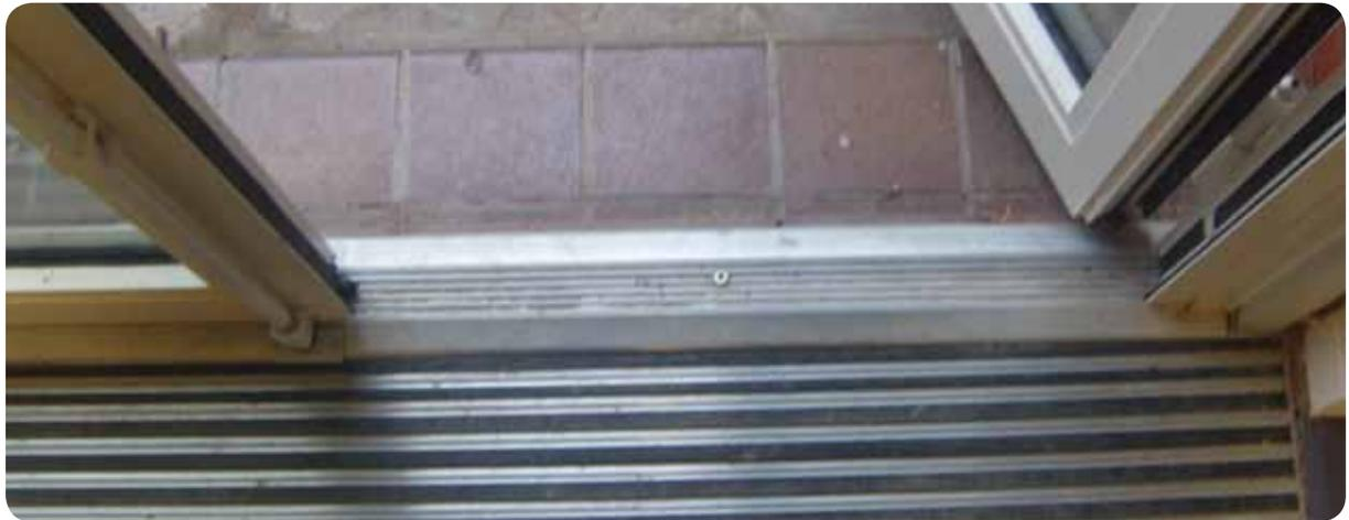
Threshold strips at entrances to buildings can often be trip hazards. They can also cause a visual barrier for people with dementia and sight loss and some individuals may not wish to cross over threshold strips. In new buildings and when refurbishing or maintaining housing we recommend level thresholds in accordance with the recommendations within Part M and BS8300 (BSI, 2010).
