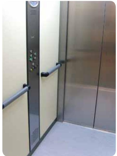
The lift incorporates a wheelchair accessible control panel.
