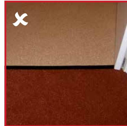
*Change in floor tone may be perceived as a step. This can be exacerbated by a contrasting threshold strip.*
