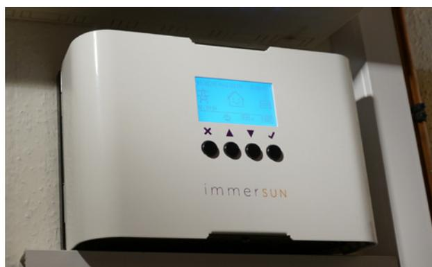
**Figure 7** Controller that enables excess solar electricity to be stored as hot water
