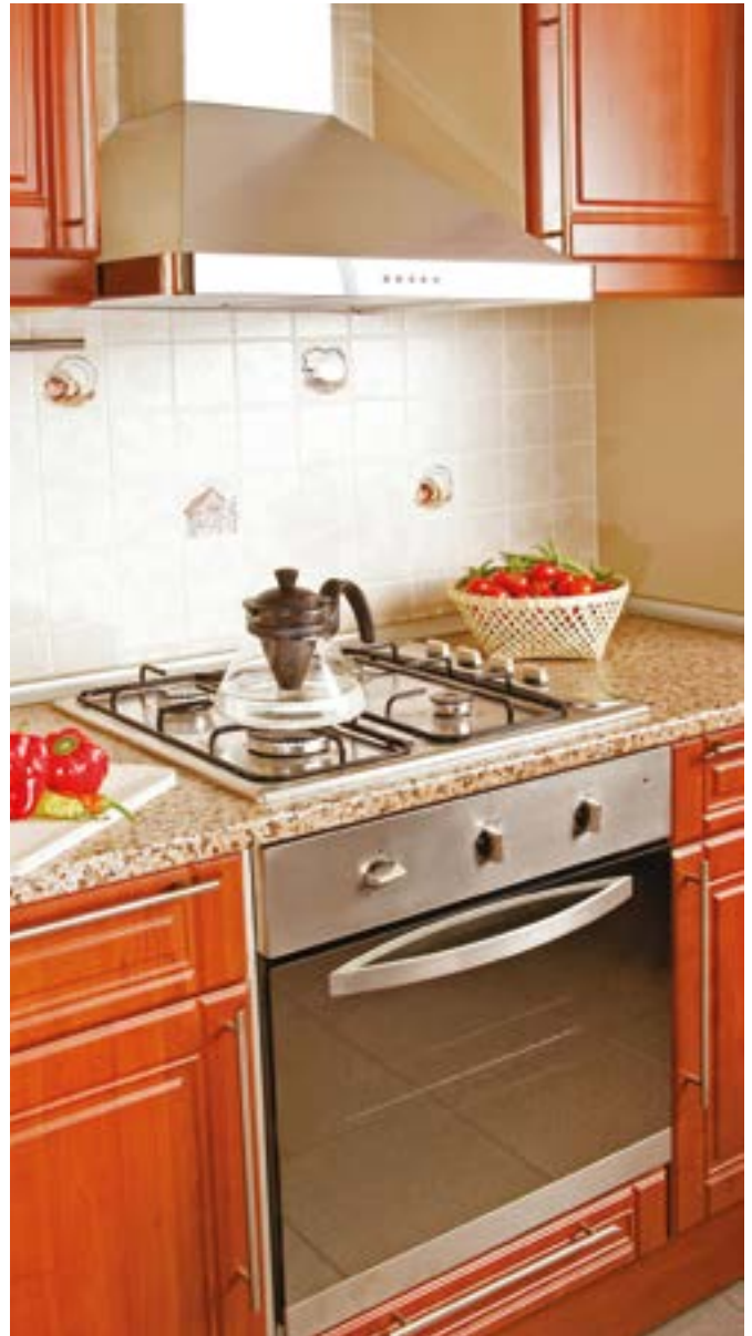
The appliances in this image are separate, with the oven placed underneath the hob ("built under")
