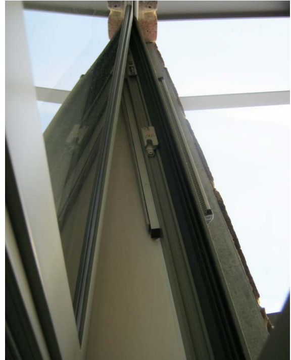
Figure 3. Trickle vents are present in all windows, and appeared to generally be in use.
