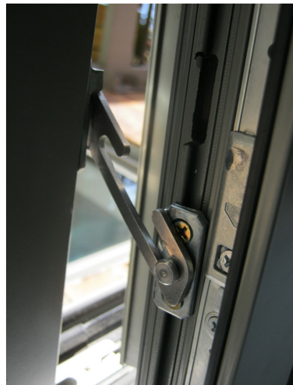
Figure 8. Restrictor in office.
