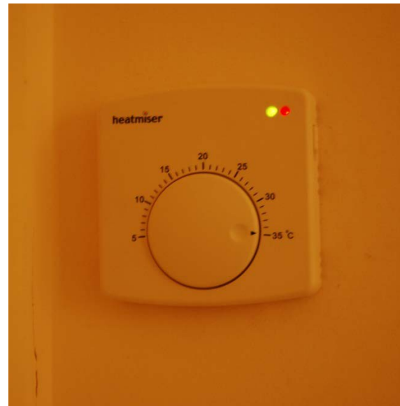
Figure 7. Room thermostat for bathroom set to 'max' due to issues with the underfloor heating. The overall heating system is left on during the summer months in case residents' require heating, and the staff have set the flat programmers to be on all day.
