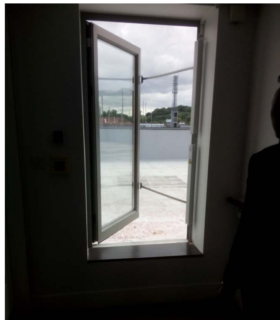
Figure 4. Flat roof with white finish increases reflectivity and thus reduces heat gain. Image also shows large windows at ends of corridors to provide additional air circulation and ventilation (note restrictors).
