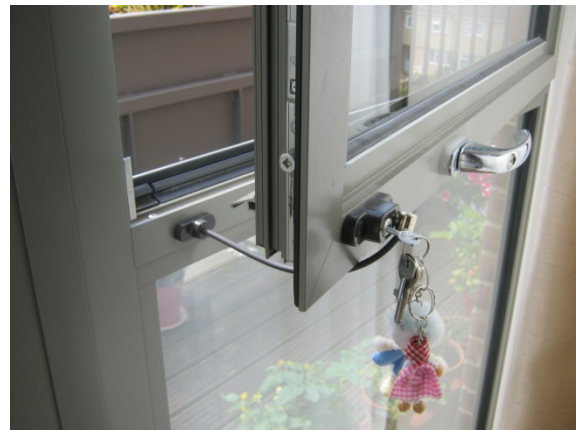
Figure 6. Window restrictors in flats have locks and can be removed if the residents want to.
