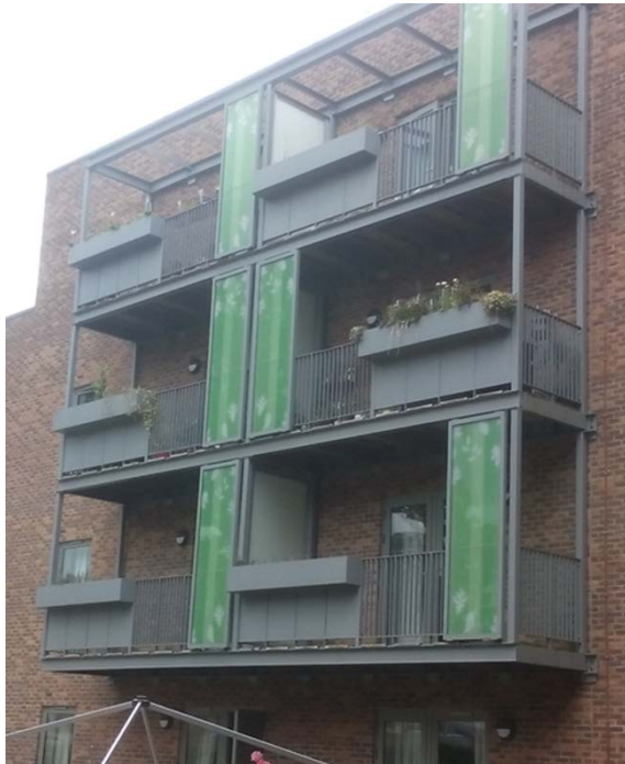
Figure 2. Wide balconies and fixed vertical panels provide additional shading to residential flats.
