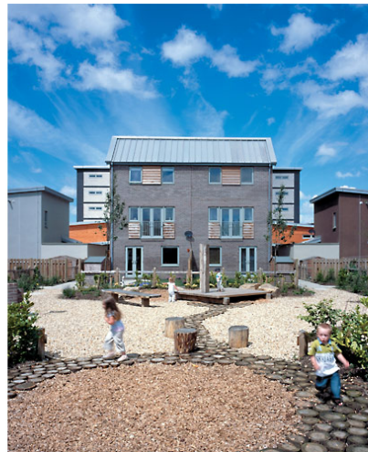
Alternative use of outside space – The Staiths Development, Gateshead
