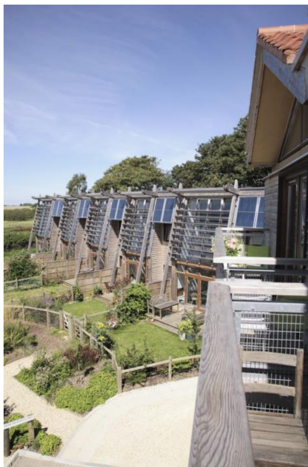
Eco Homes Scheme, Great Bow Yard, Somerset demonstrating sustainable construction.
