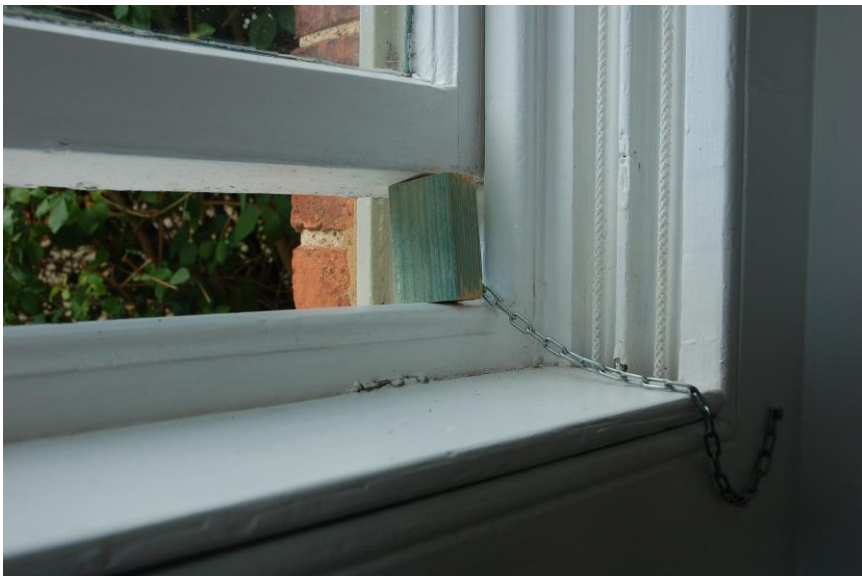
Figure 13: Window propped open by staff in case study B using block of wood to provide fixed air flow
