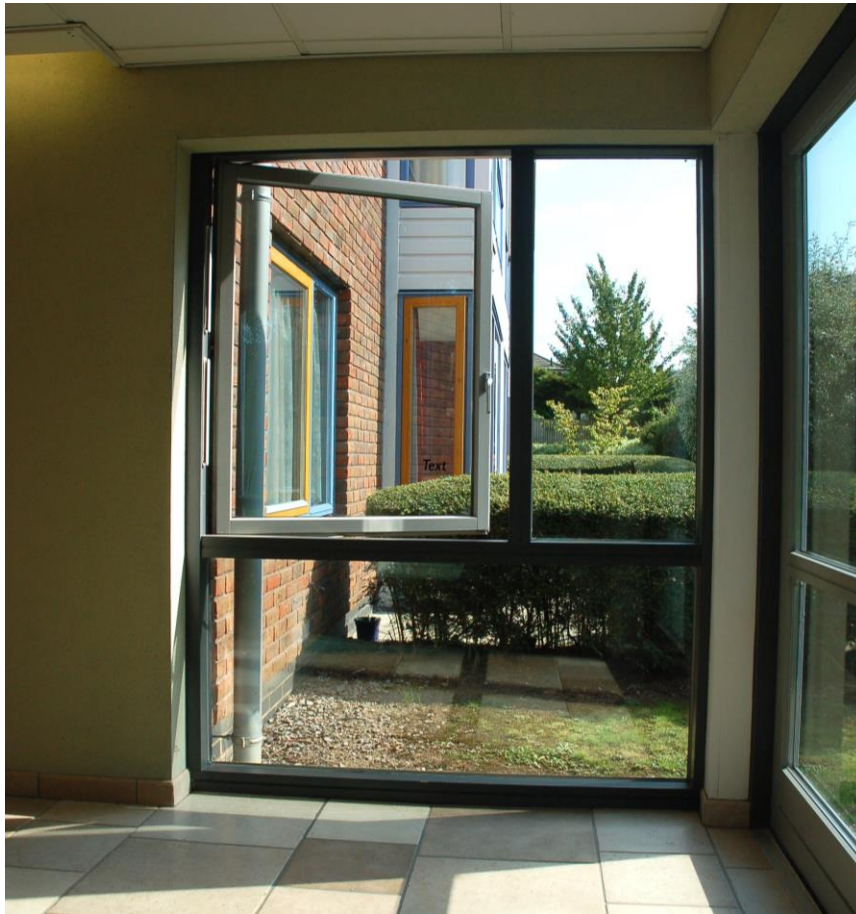
Figure 9: Corridors with large opening windows provide cross-ventilation throughout communal spaces (as well as for flats/bedrooms)
