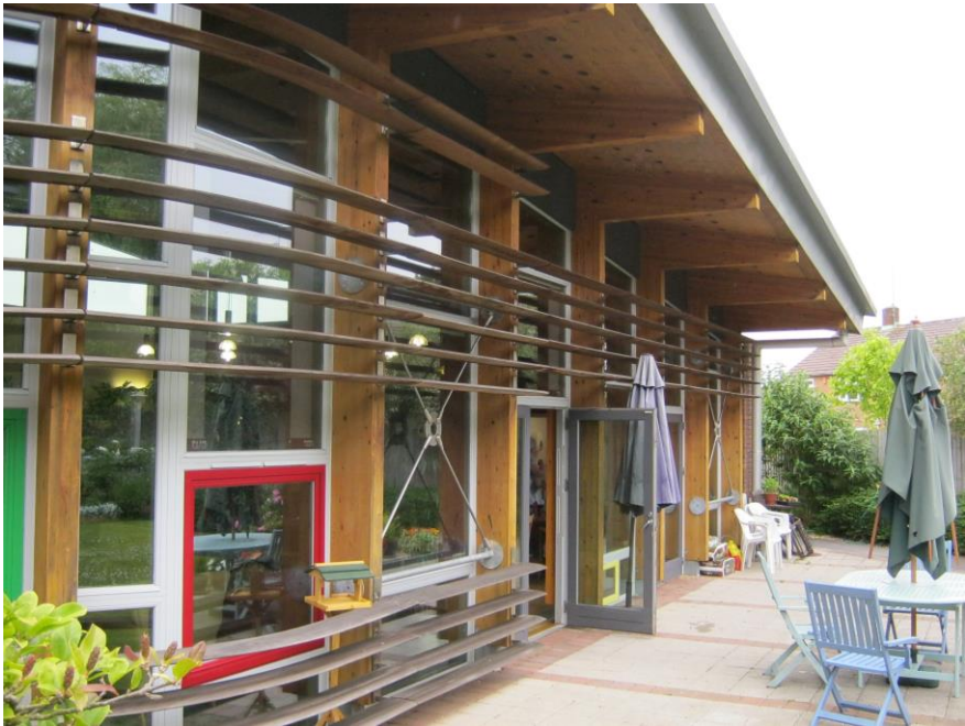
Figure 8: Deep balconies in case study D provide additional shading to rooms below
