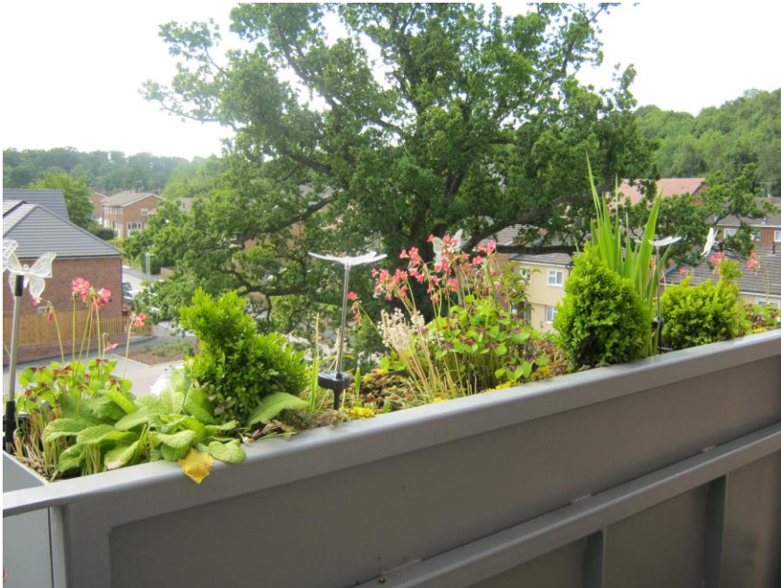
Figure 6: Built-in planters on balconies provide additional vegetation to assist with cooling
