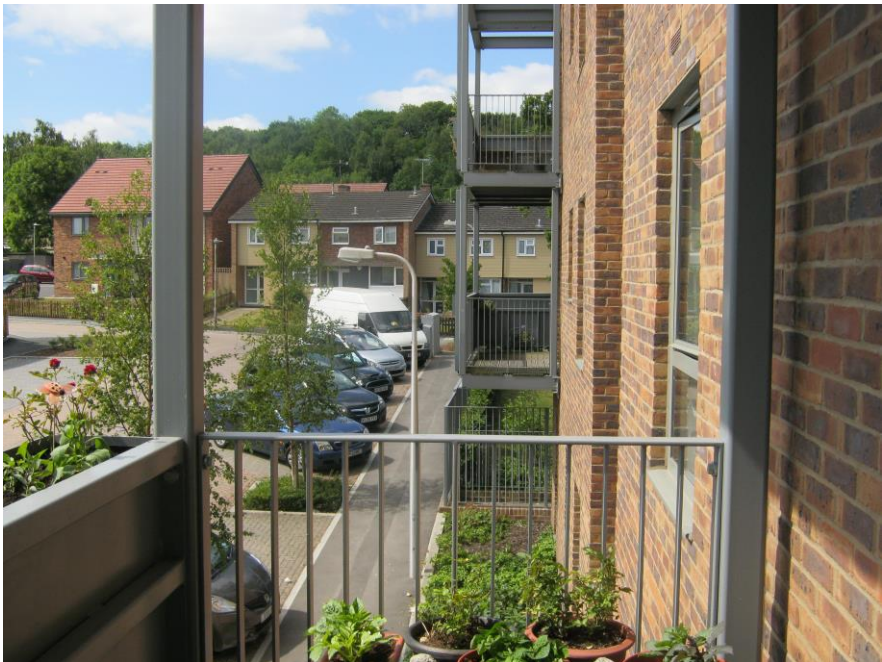
Figure 8: Deep balconies in case study D provide additional shading to rooms below
