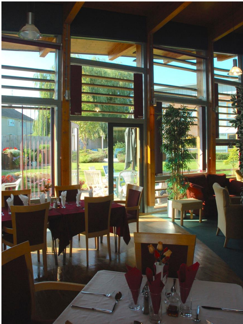
Figure 1: Minimising heat gain through use of external fixed shading (brise-soleil)
