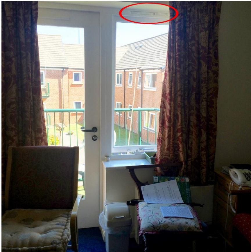
Figure 11: Trickle vent above window in bedroom cannot be opened due to being painted over and sealed closed
