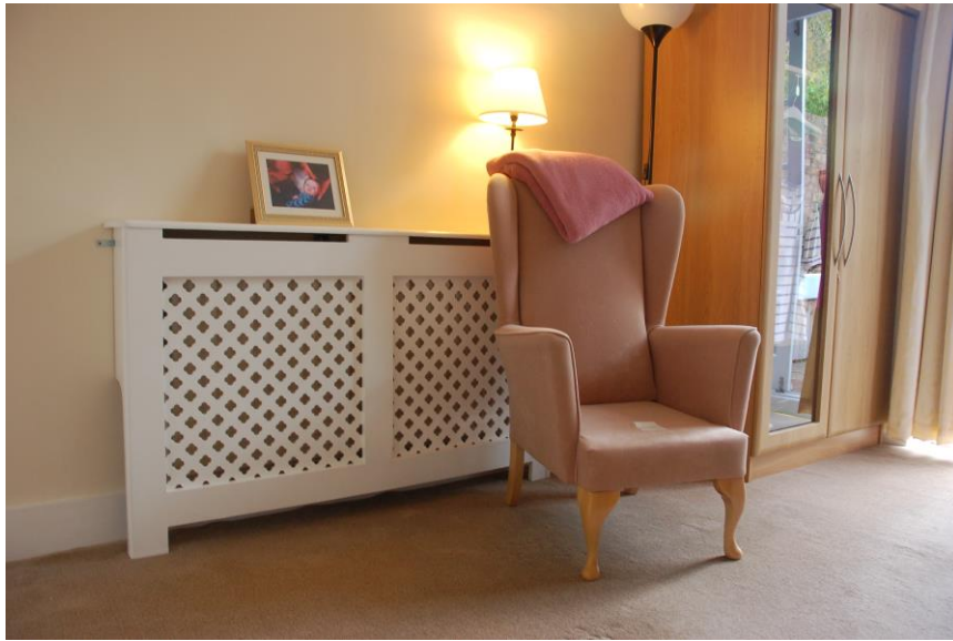
Figure 10: Radiators covered to prevent residents' access in case study B
