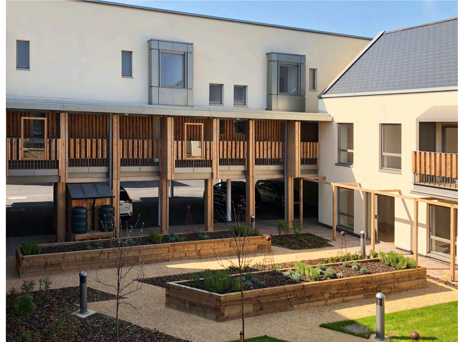
Steepleton - Retirement Community in Tetbury
