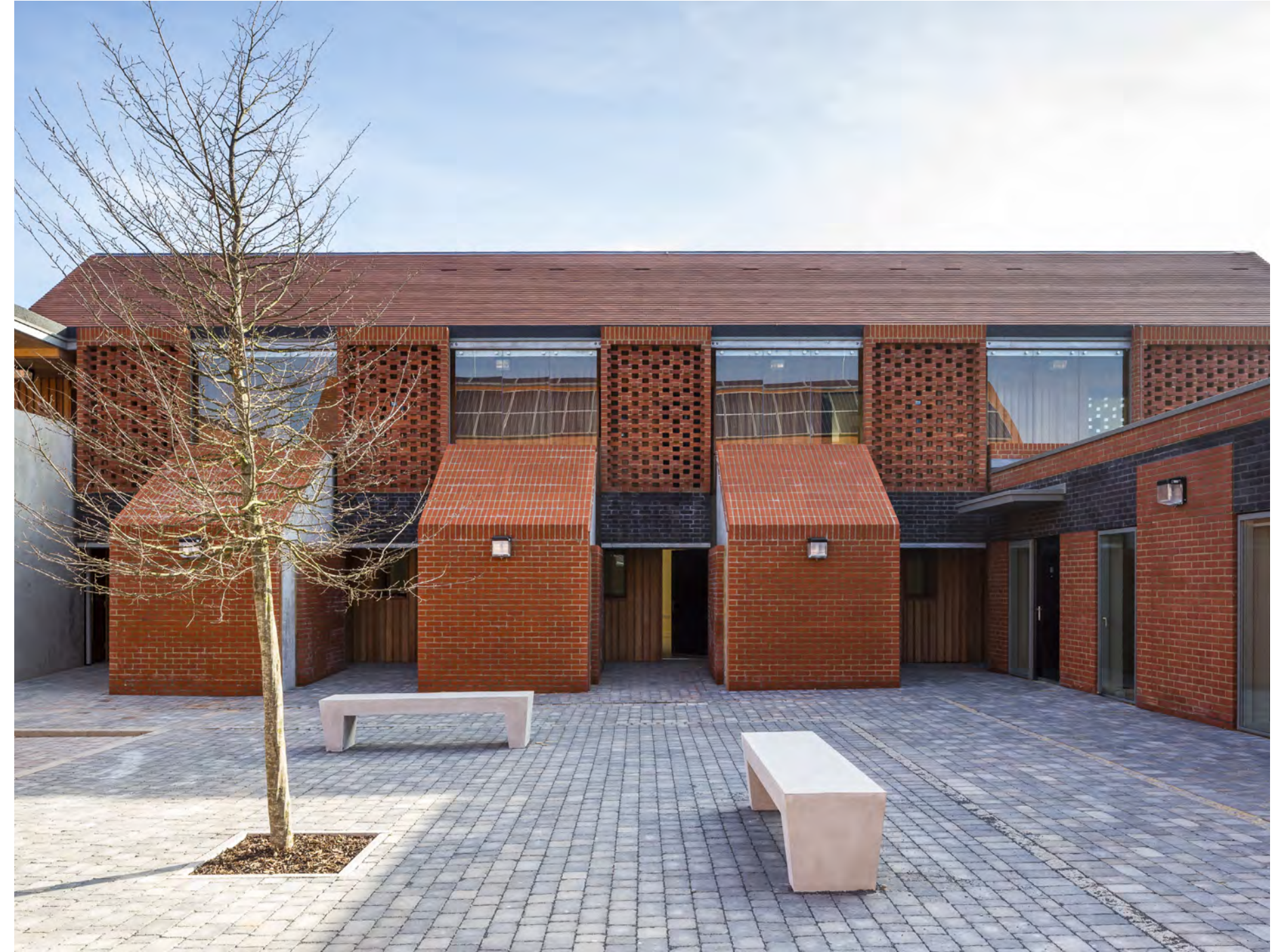
Hargood Close - Accommodation for the homeless in Colchester
