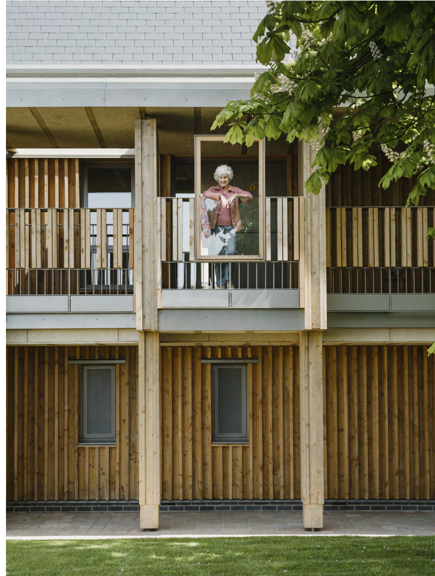
Steepleton - Retirement Community in Tetbury
