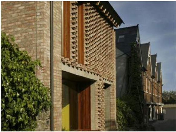
Protruding brick wall example
