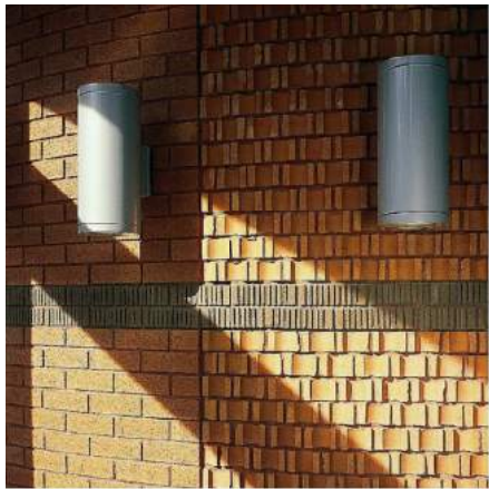
Cut header brick facade
