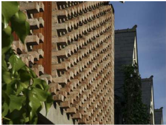
Protruding brick wall example
