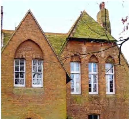
Simple brickwork detailing.
