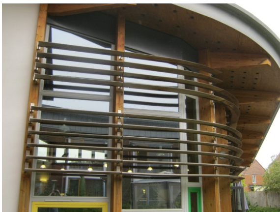
Figure 2. External brise-soleil and large overhanging eaves on building façade to main communal lounge area.
