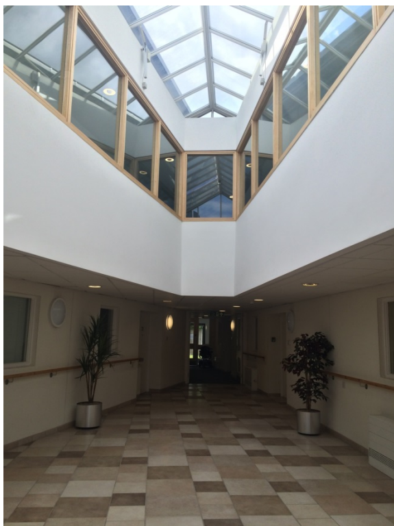
Figure 6. Openable rooflights in communal areas provide opportunity for stack ventilation.
