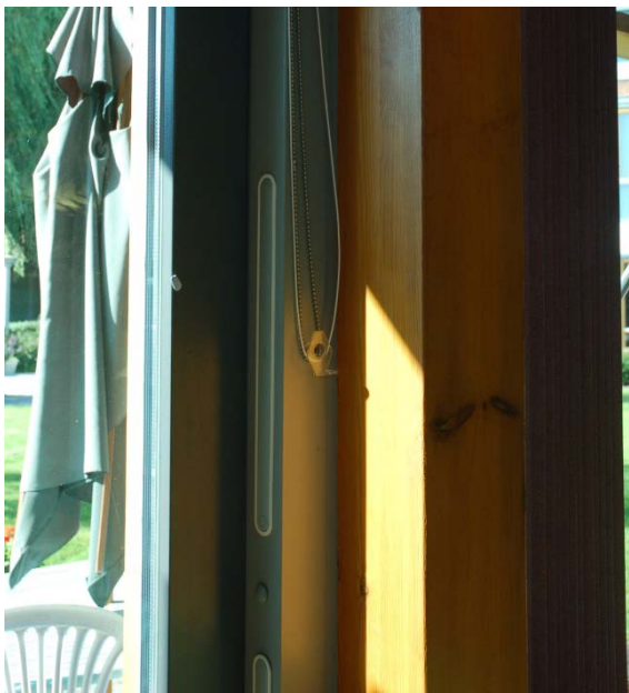
Figure 3. Trickle vents installed on all windows.
