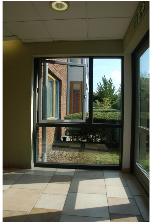
Figure 4. Cross-ventilation in communal areas provided by openable windows at sides and ends of corridors.
