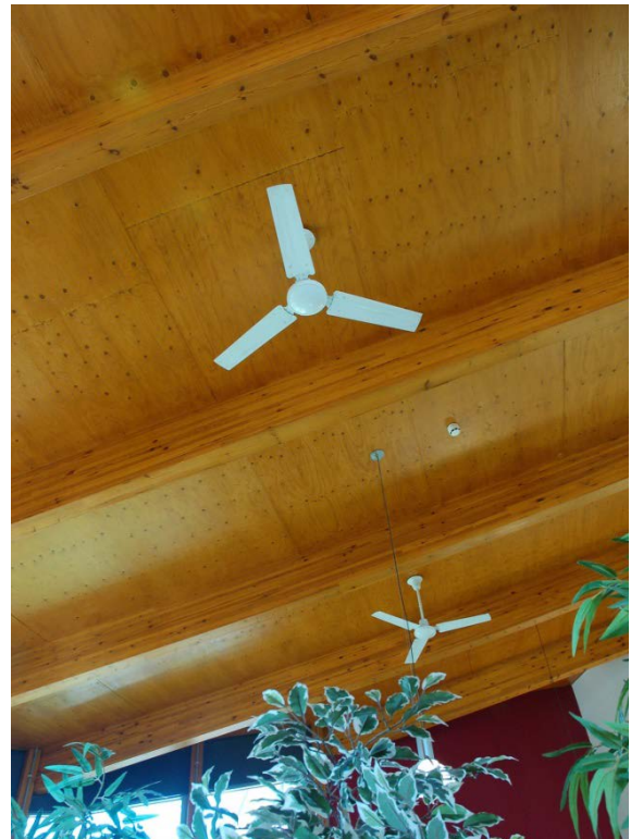
Figure 5. Fixed ceiling fans installed in main communal lounge to provide additional air circulation during periods of hot weather.
