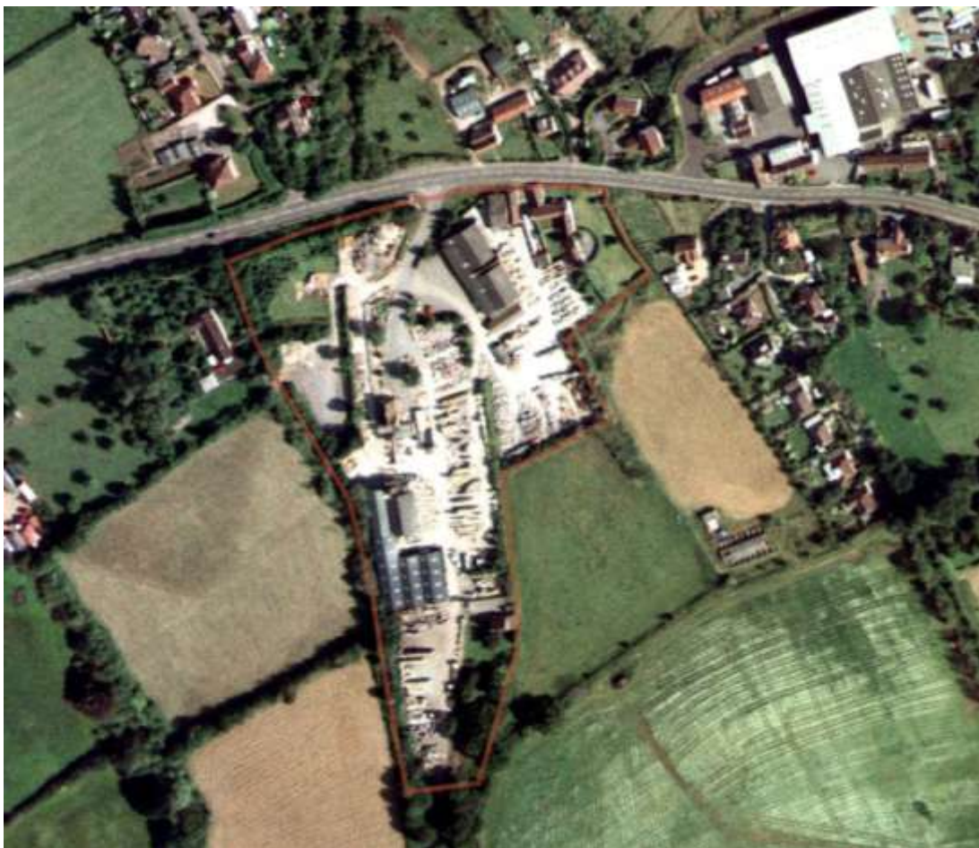
Figure 6.10: The former employment site at Sandford Station
