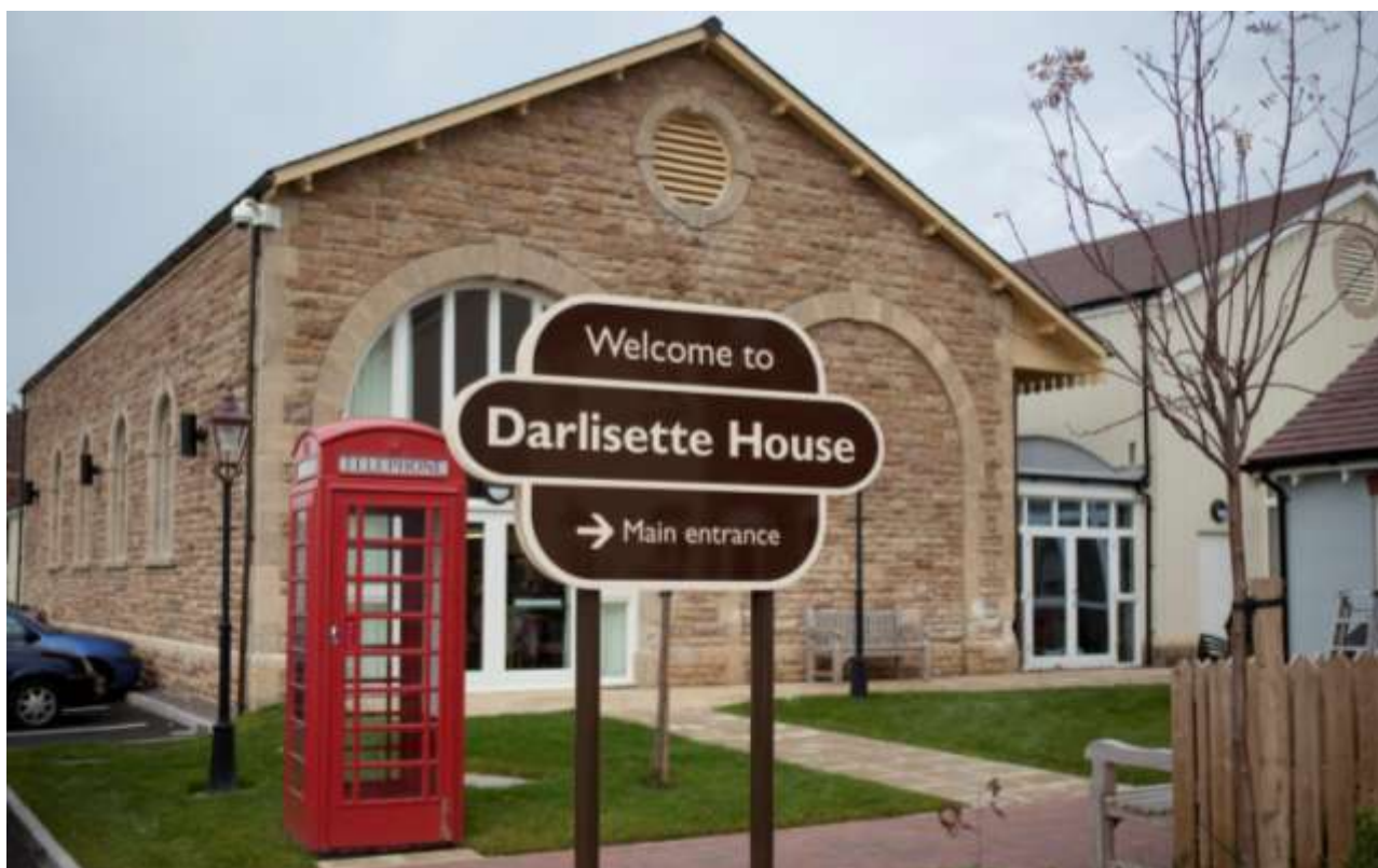
Figure 7.5: The community building at Sandford Station, designed to combine the historic character of the existing buildings on site with the need for modern housing and care facilities
