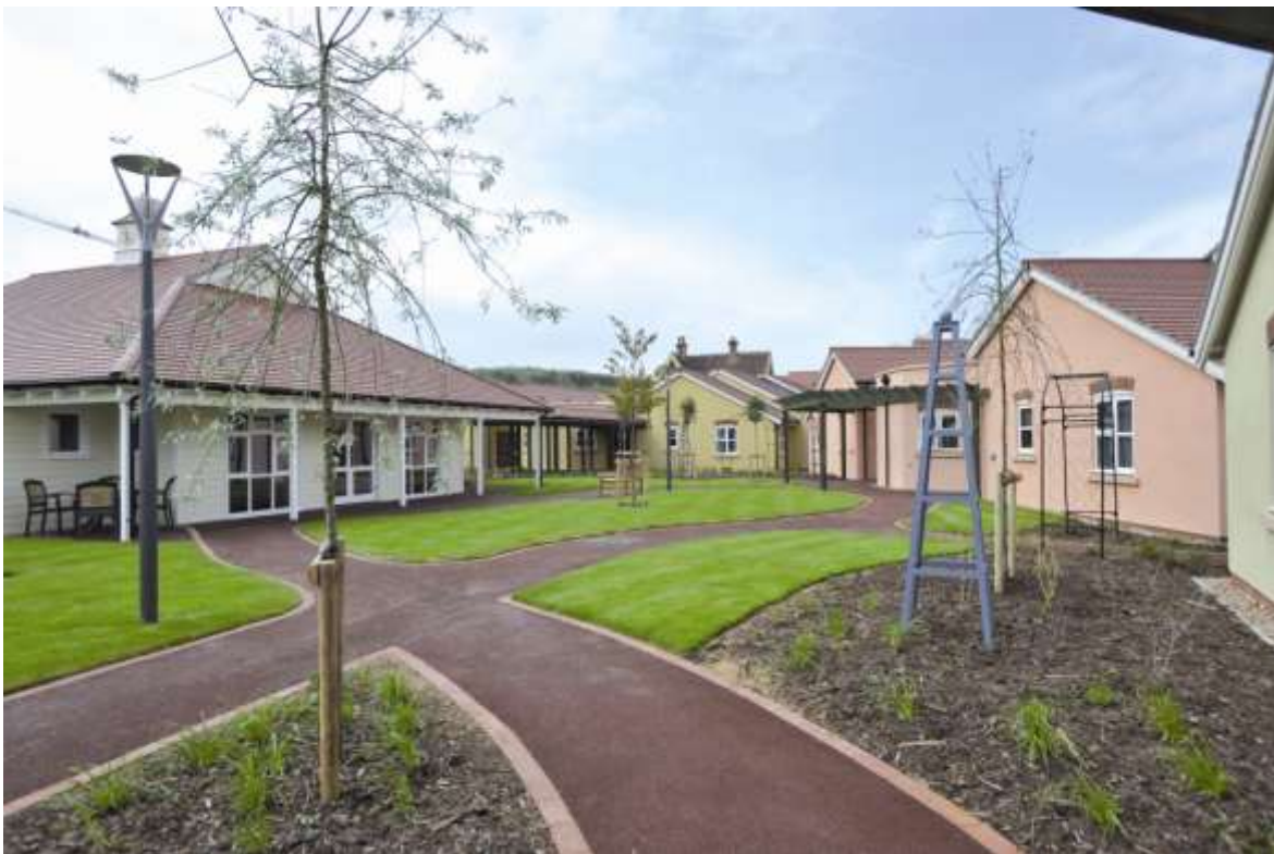
Figure 8.2: Dementia care accommodation at Sandford Station. Such provision of accommodation with care fails to be acknowledged in the majority of development plan documents
