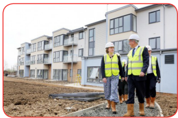
Site of Weaver's Court, Alnwick
