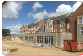
Construction work at Herriot Gardens, Sowerby
