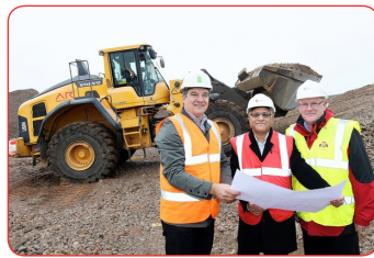
Site work on the new scheme in Loughborough
