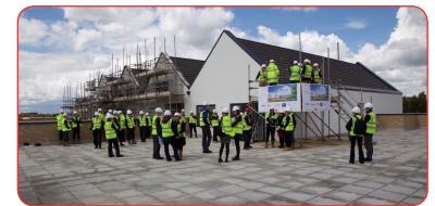
Construction at the new care village in Bowthorpe
