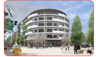
Bournville Gardens retirement village, Birmingham
