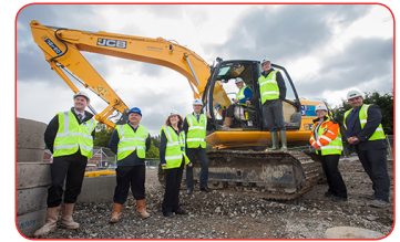
Work at the construction site in Powys
