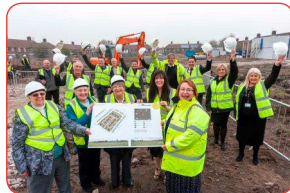
On site work at the new scheme in Dovecot
