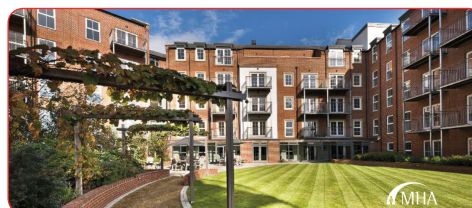
Welland Place in Market Harborough
