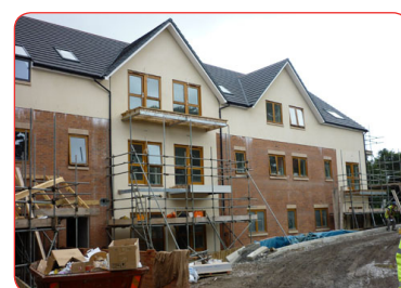
Llys Jasmine Extra Care Housing scheme under construction in Mold, Flintshire in Wales
