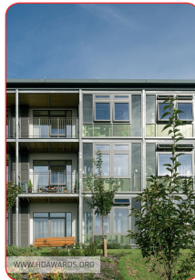
Prince Charles House, St. Austell
