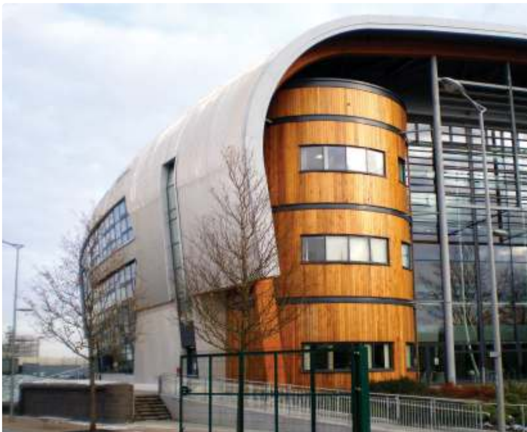
South Bristol Skills Academy – health services need to be involved in the local authority's infrastructure planning process
