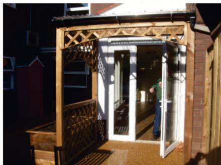
Porch with clear roof, handrail and raised bed
