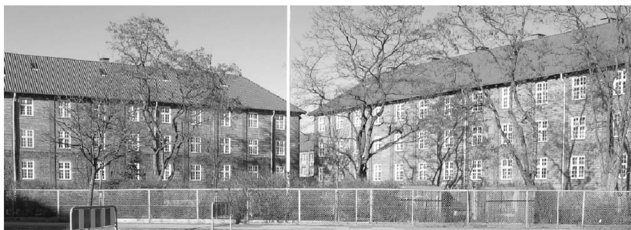
Figure 3. Engholmen Nord housing estate in Copenhagen
