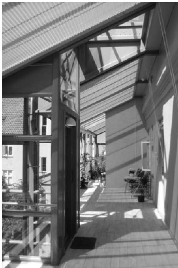
Figure 6. Another urban renewal demonstrations project where broad recreational balconies and an elevator were built outside the facade of an existing building. In this case one elevator gave access to more staircases. ( http://www.paalsson.dk/ )
