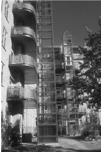
Figure 5. Urban renewal demonstrations project where small balconies and an elevator have been installed. The elevator was installed because new flats were made in the attic. Thereby also the other flats got access by an elevator. ( http://www.paalsson.dk/ )
