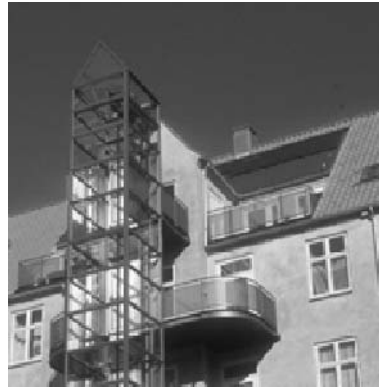
Figure 5. Urban renewal demonstrations project where small balconies and an elevator have been installed. The elevator was installed because new flats were made in the attic. Thereby also the other flats got access by an elevator. ( http://www.paalsson.dk/ )
