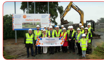
Development work on Hafan Cefni, Llangefni
