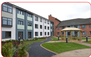
Brooklands Gardens, Market Harborough
