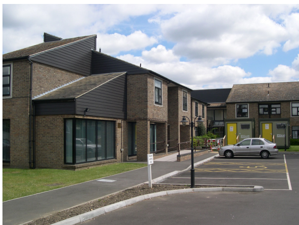
The original building prior to demolition – note the Portacabins installed to accommodate temporary plant to deal with issues arising from failing M&E services
