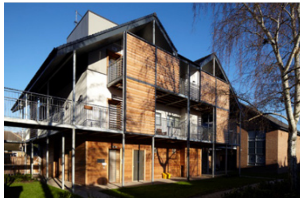
View of the central block from the communal garden showing the lift on the left hand side
