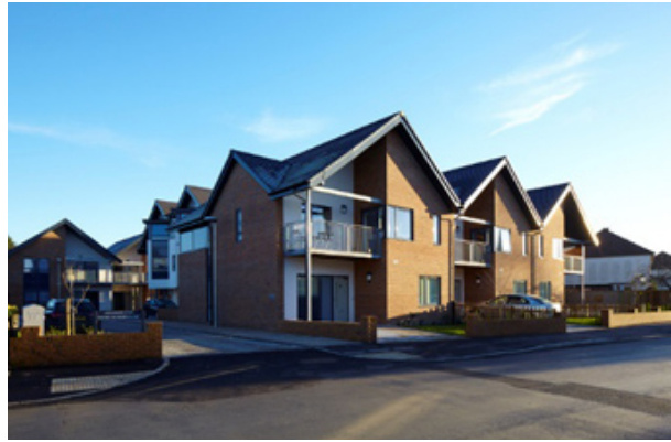
View of Castlemaine Court from Rectory Lane
