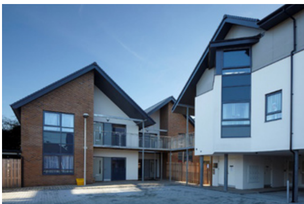
View of parking area, central 3 storey block and privacy fence controlling access to the flats and communal gardens
