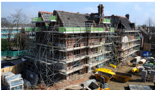
St Bedes in Bedford, under construction
