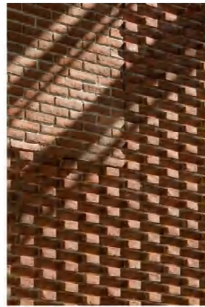
Protruding brick wall example using similar coloured brick to those intended on the west block
