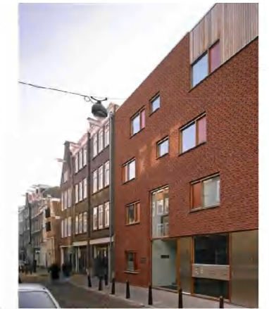
Example of facade with exposed 'frogs' with the top of the brick facing out
