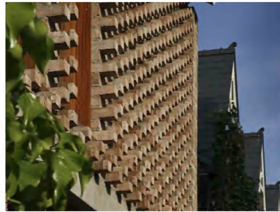
Protruding brick wall example
