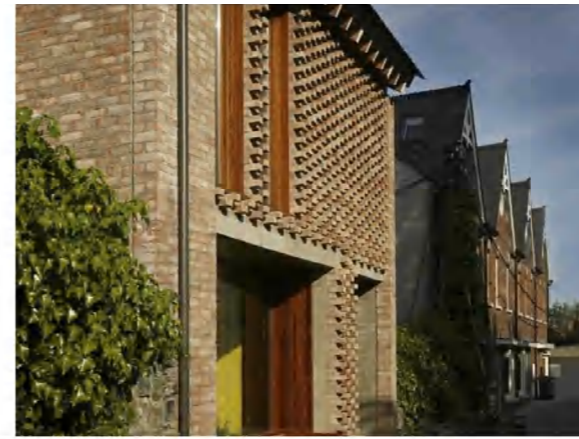
Protruding brick wall example
