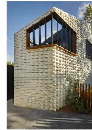
Protruding brick wall example using similar coloured brick to those intended on the east block
