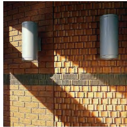
Cut header brick facade
