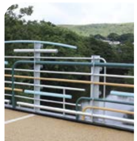
Clydach Cycle Route
