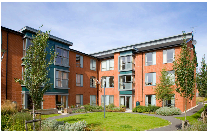
Showell Park, Wolverhampton (SIPS construction for Senior Living Housing)
