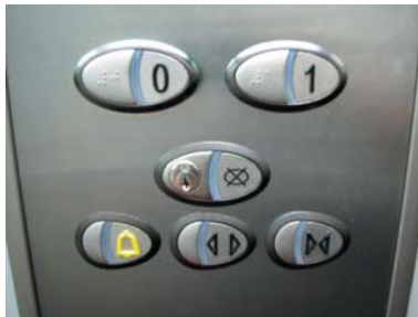
Large, legible and tactile buttons to lift panel
