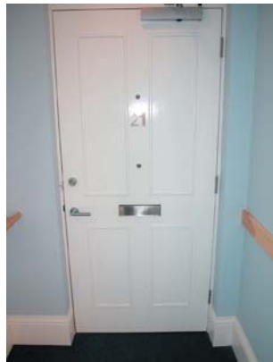
Flat entrance door showing twin-spyholes and free swing close
