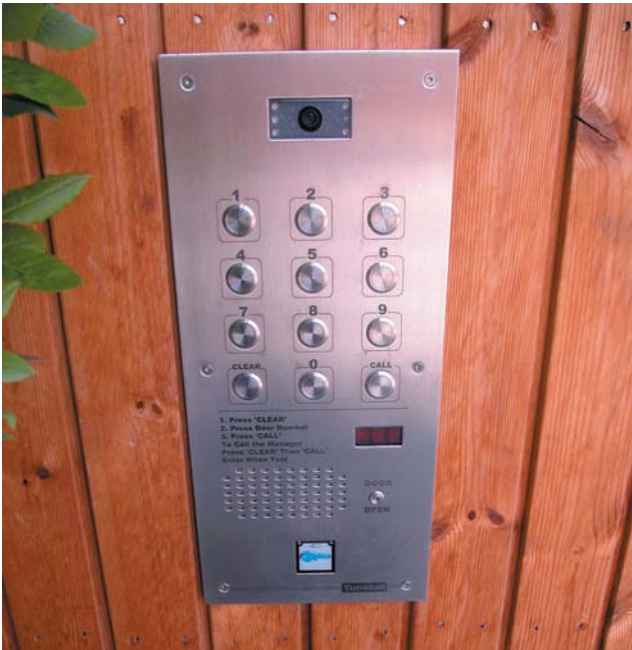
Integrated entry panel with key-fob reader, CCTV and speech
