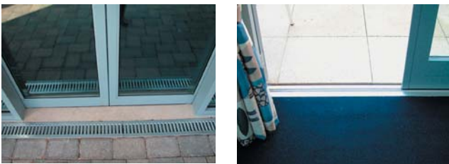
Flush threshold, main entrance and entrance matting.
