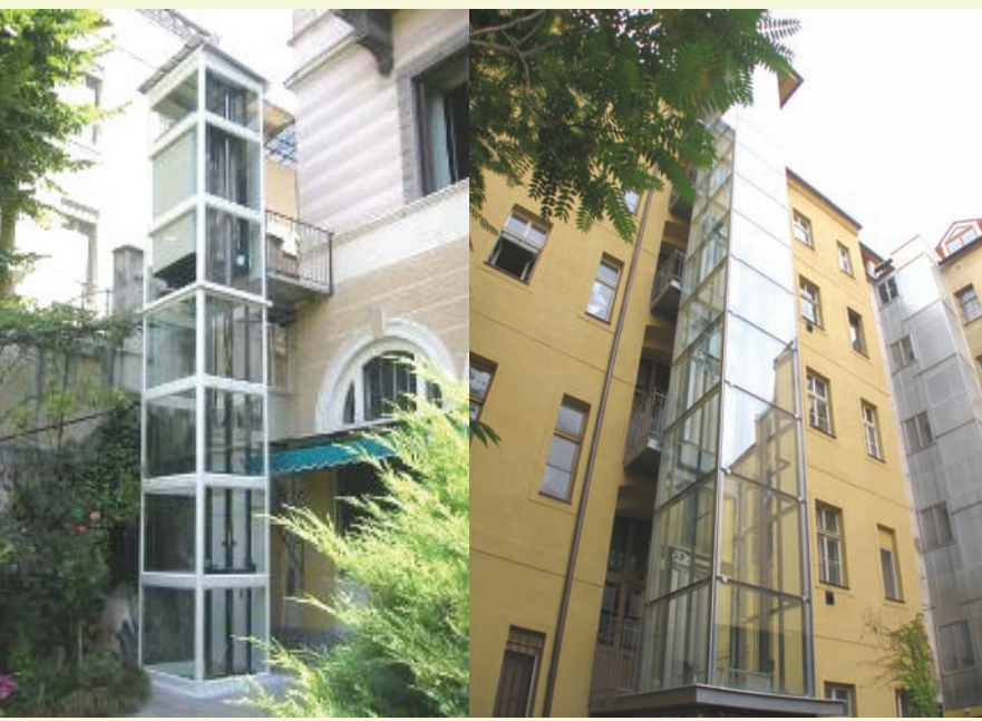
images of lifts positioned on the outside of the building
