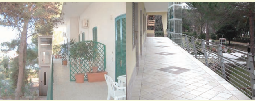
cases of lifts installed in a gallery typology
