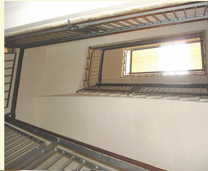
wide stairwell in which to install a lift
