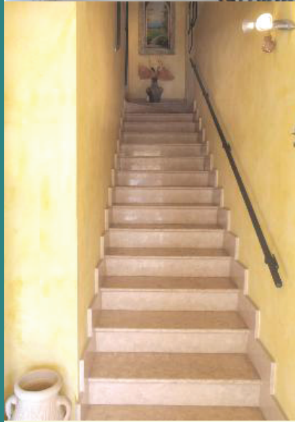
images of buildings with insufficient stair wells for the positioning of lifts
