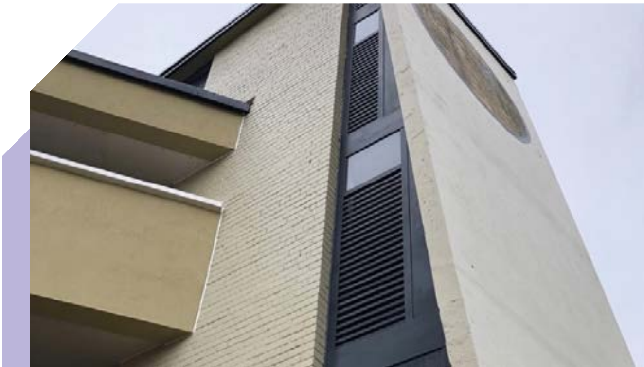
Stairwell exterior following improvement works, 2019
