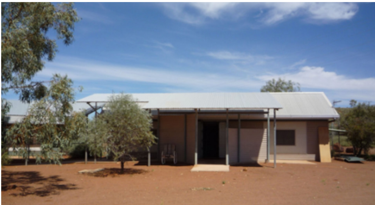
One of the small buildings of TPN
