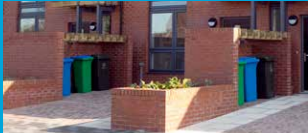
A good example of bin storage
