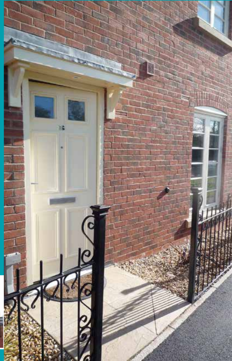
This window pattern suits the materials used in the wall
